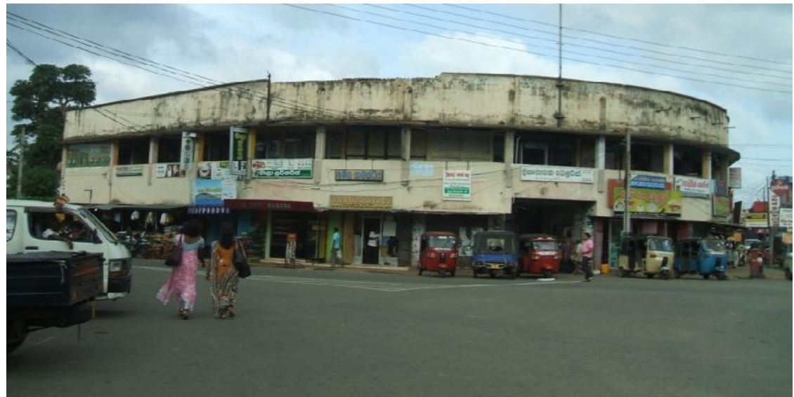
Existing Market Building
